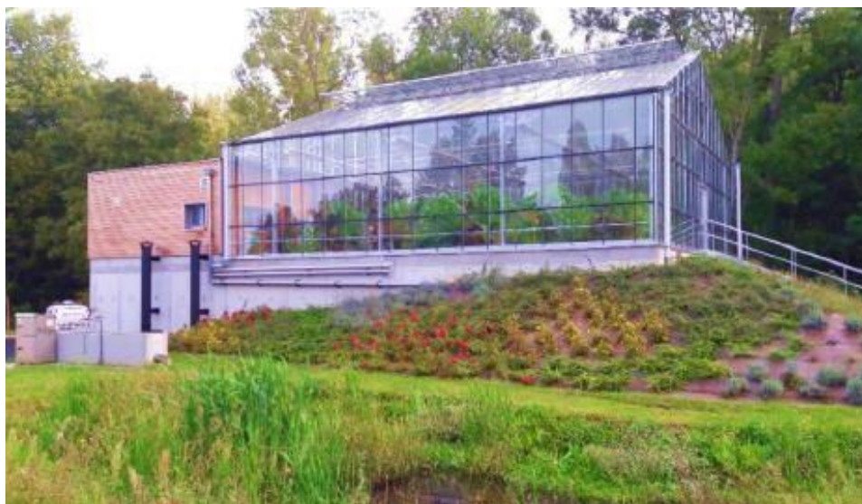
Figure 14 : Station Organica de Nogent-sur-Vernisson (41) - 3 500 EH
